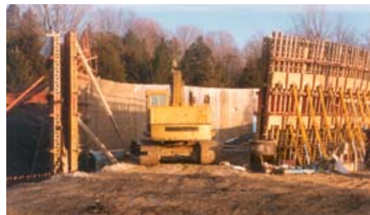
Concrete forms ready to pour the Visitors Center
